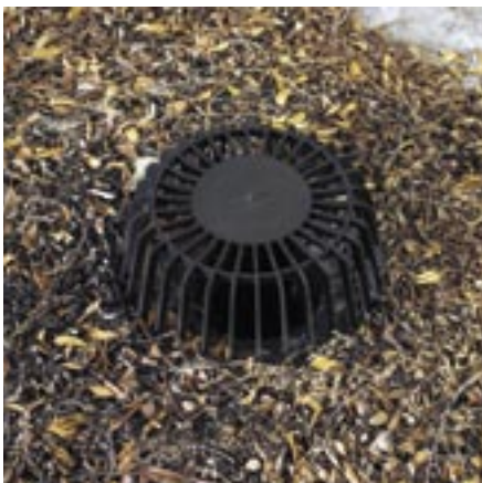
Clogged drainage openings
